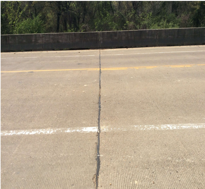
PHOTO 1 Description Bent 6 joint material is beginning to loose contact with the concrete, this is typical of all joints.
