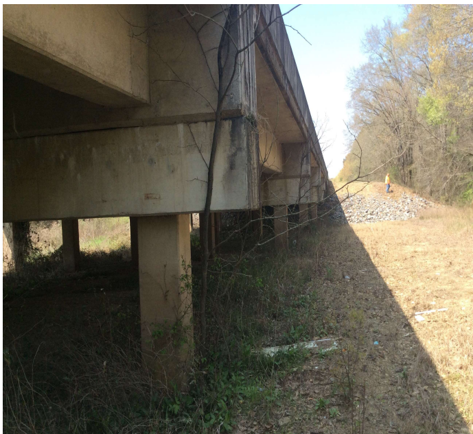
PHOTO 3 Description Bent 5 looking back, minor vegetation growing under & up beside the bridge.
